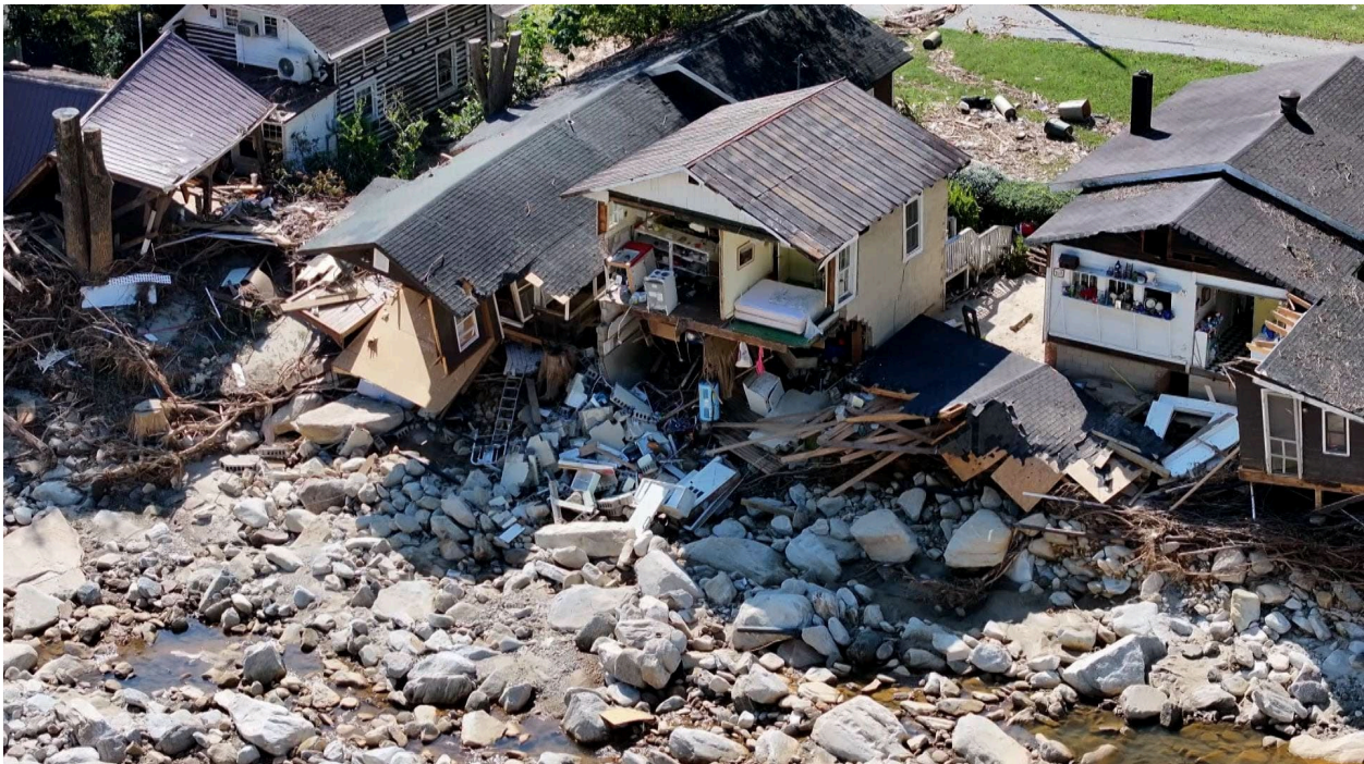
Home damaged by the Broad River in the town of Chimney Rock. (Rutherford County, North Carolina)
