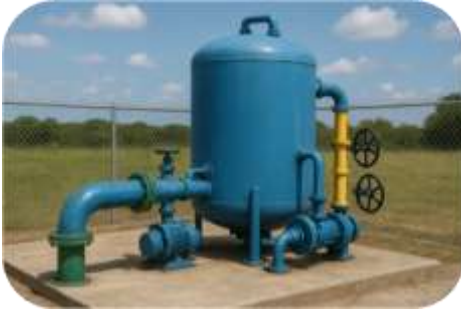
A building project?
